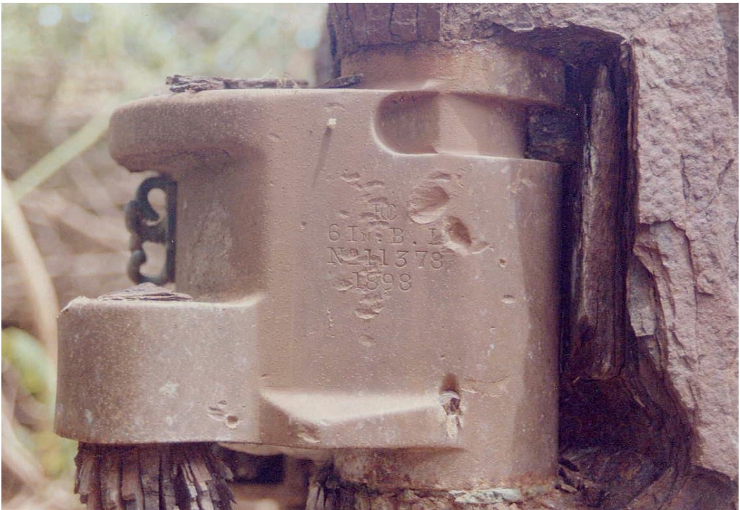
Figure 6. Breechblock of a Elswick Ordnance Company 6-inch gun on Taroa I., Maloelap Atoll
