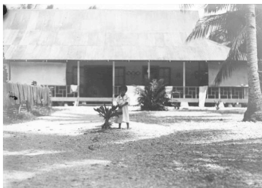
Figure 5 : Main House after Iron Roof Installed – c. 1915; Photo: De Brum Collection, Alele Museum, Majuro; with permission Leonard De Brum
